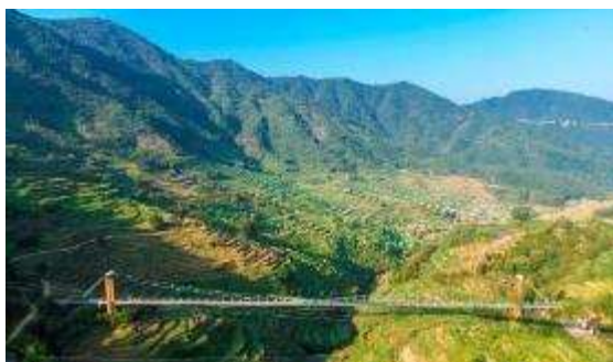
Wuyuan Glass Bridge
